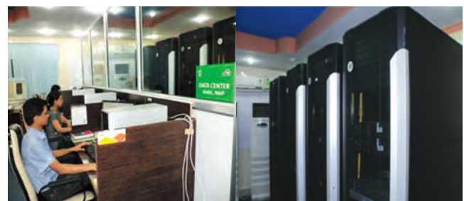
HPC Infrastructure at NBAIM, Mau
